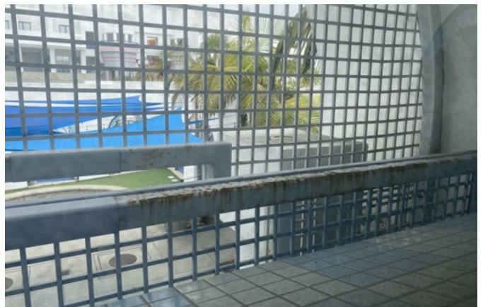
Exterior arch on east building façade
