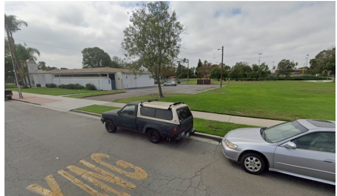
John Landes Community Center Library Exterior
