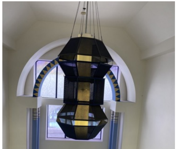
Existing suspended pendant light fixture with painted mesh cages
