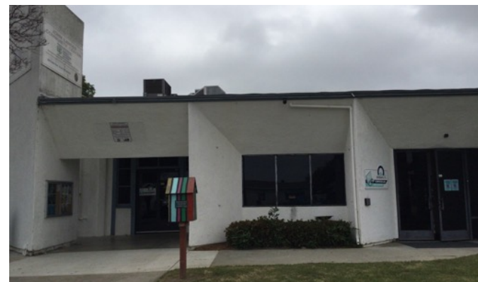
Two sets of main entry doors from Cedar Road
